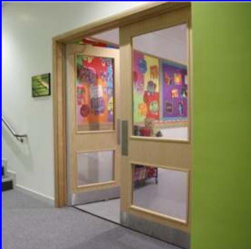
**Guardian Finger Safe** offers finger and hand protection with a built in guard on the hinge edge of the door
